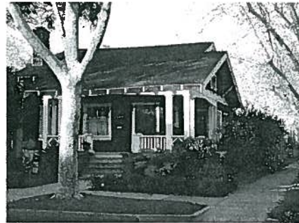
Figure IIIA-1a1: Entry porch highlights primary entry to the house and is oriented toward the street
