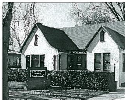
Figure III B-5c: Building is divided into smaller component parts to reduce perceived mass
