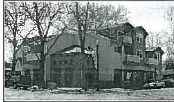
Figure III B-4b: By stepping back upper stories and using similar roof patterns, this building does not look massive in a predominantly single-family neighborhood
