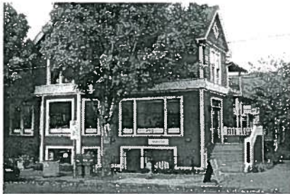
Figure III B-3a: The front/primary entry to this building is clearly defined by raising it above the driveway level
