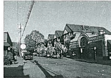
Figure III B-5b: Front elevation of a Horizontal Residential Mixed-Use in a Single-Family Neighborhood
