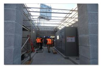
The walls for new solids handing building and sludge thickener are now complete and sludge tank top and building roof are being formed.
