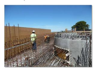
The Electrical building walls have been completed. Electrical panels have been craned in through the open roof and are now being sealed in.
