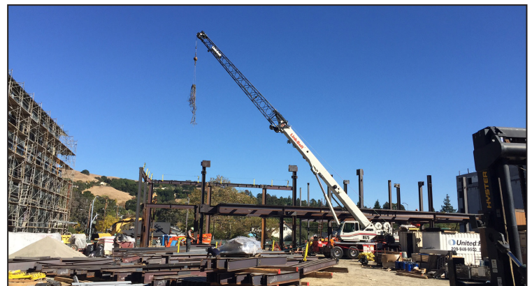
Library Building Steel Erection
