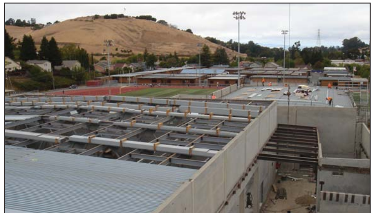
Gymnasium Building E Roof Decking and Lobby Steel
