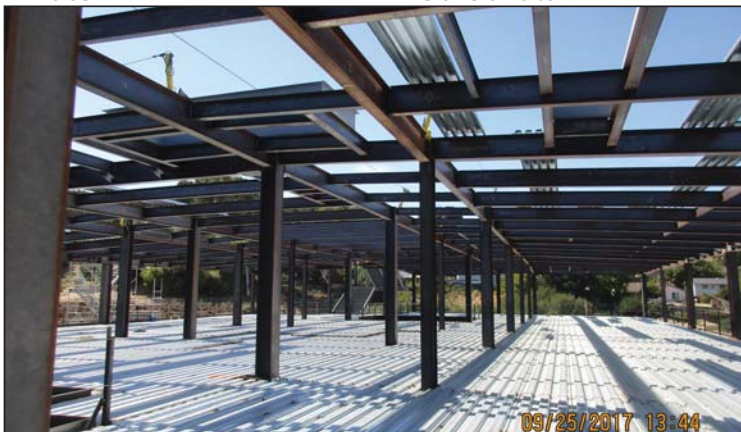
Classroom Building D Structural Steel Decking
