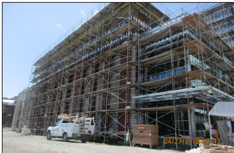
Classroom Building Brick Veneer and Storefront Windows Installed
