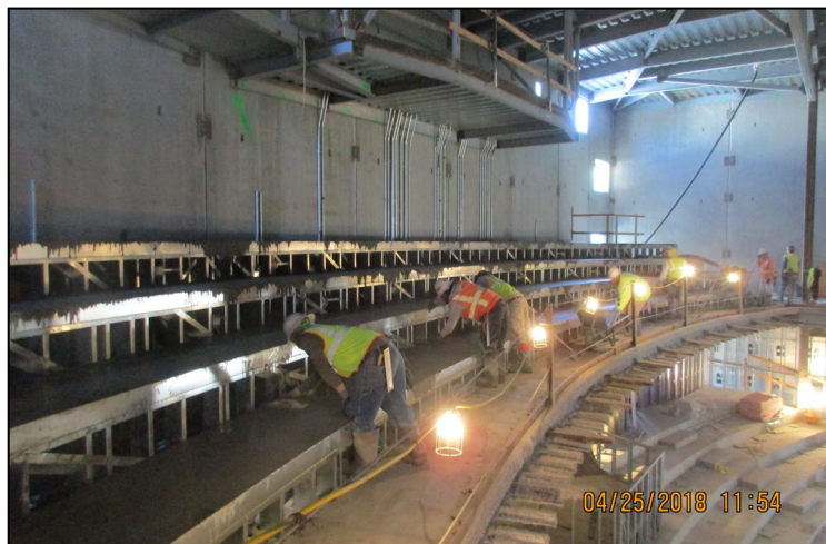
Concrete Pour of Framed Seating Decks on Theater Balcony
